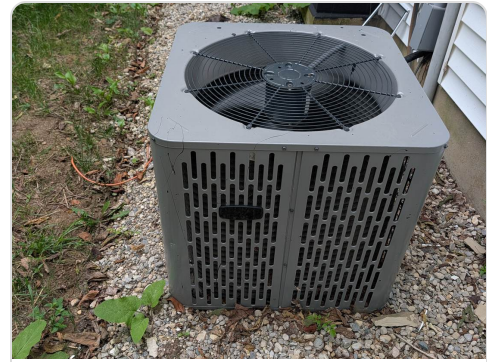
Equipment schedule · labels from the walk
